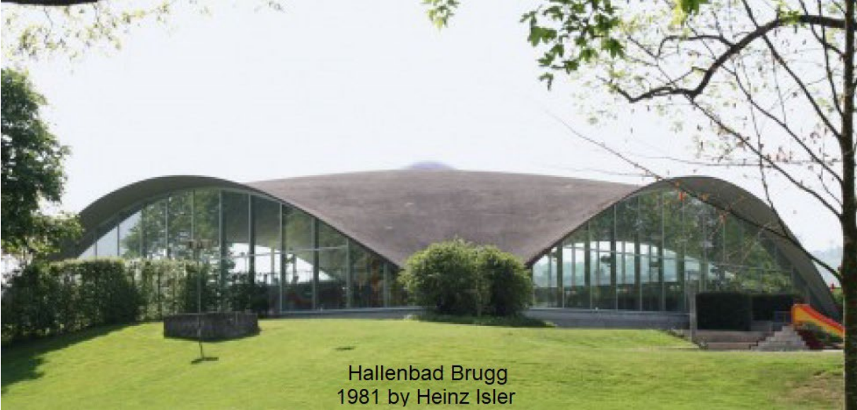
Figure 64 Hallenbad by Heinz Isler [image Peter Eigenraam]
